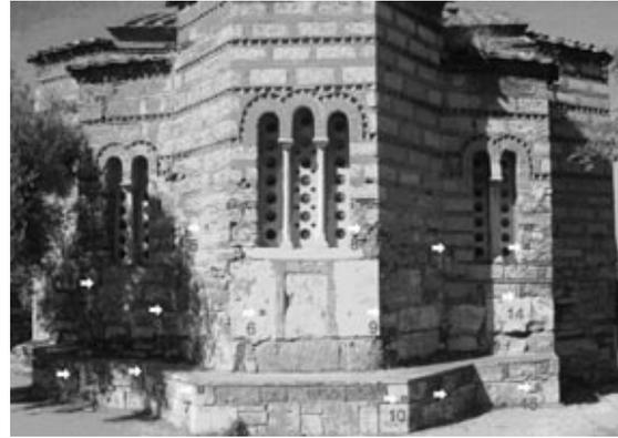
Figure 7: Target positions measured on the façade
